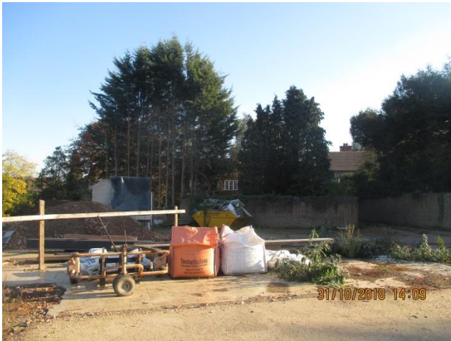
View of site facing southern boundary and view of access into site
